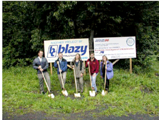
Pictured left to right: AVTEC Director Fred Esposito, DOLWD Assistant Commissioner Guy Bell, AVTEC Connected Education Department Head/Instructor Debra Burdick, DOT&PF Public Facilities Branch Project Manager Kim Mahoney and Blazy Construction Project Manager Randy Nelson.
