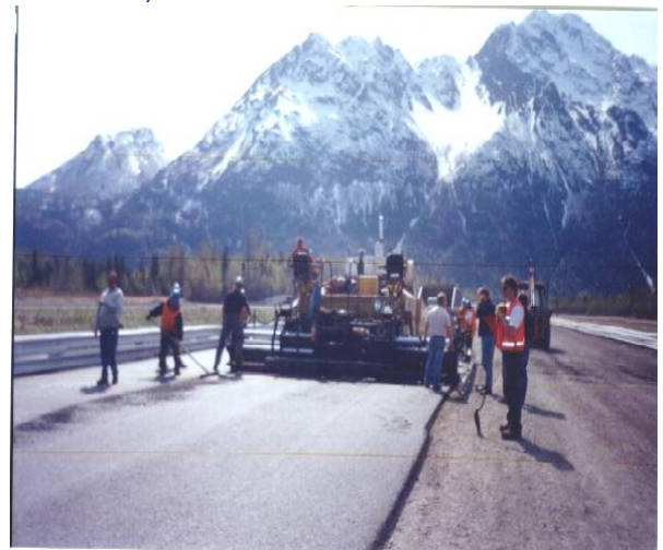
STEP, Road Builders under Construction
