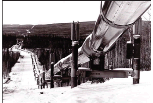
Civil engineers helped design and construct the 800-mile Alyeska Pipeline, shown near Livengood in this 1959 Alyeska photo. The pipeline crosses three mountain ranges and more than 800 rivers and streams. Soil that shifted due to permafrost was just one problem engineers had to solve during construction.
